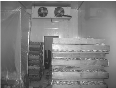
图 3 湿冷通风库贮藏柑桔 Fig.3 Citrus store in the ventilating storehouse with refrigerating and wetting systems
